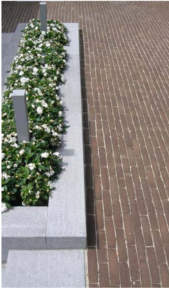
Image 5. Example of Portland stone edging and SeptimA clay pavor
